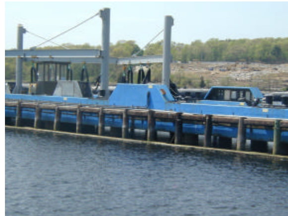
Figure 2 – Timber Fender System
